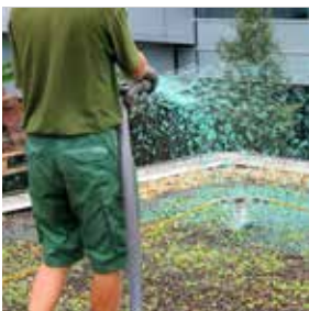
ND Hydroseeder - spraying emulsion layer on top of the ND Sedum Cuttings
